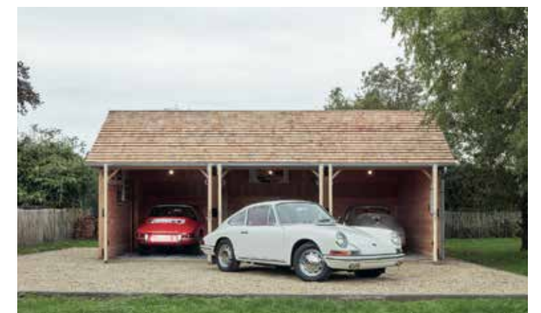
8-10 Houtbouw Defreyne (Ardoois, B), wooden triple garage, Ternat (B), 2020
